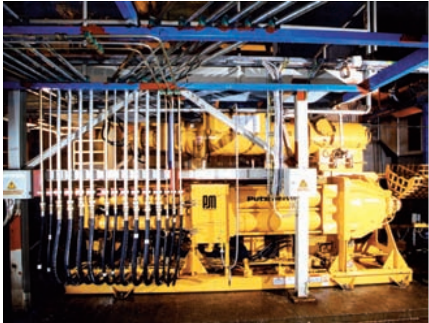
High-density solids pump in Jaworzno Power Plant, Katowice/Poland
